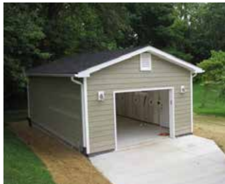
2) A larger structure that is between 200-720 square feet would be required to be similar to the main structure. A similar color of siding would meet this requirement.
